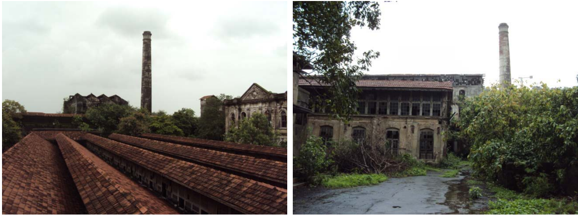
Figure 64 : Mill premise, Figure 65: Mill premise (Author)
