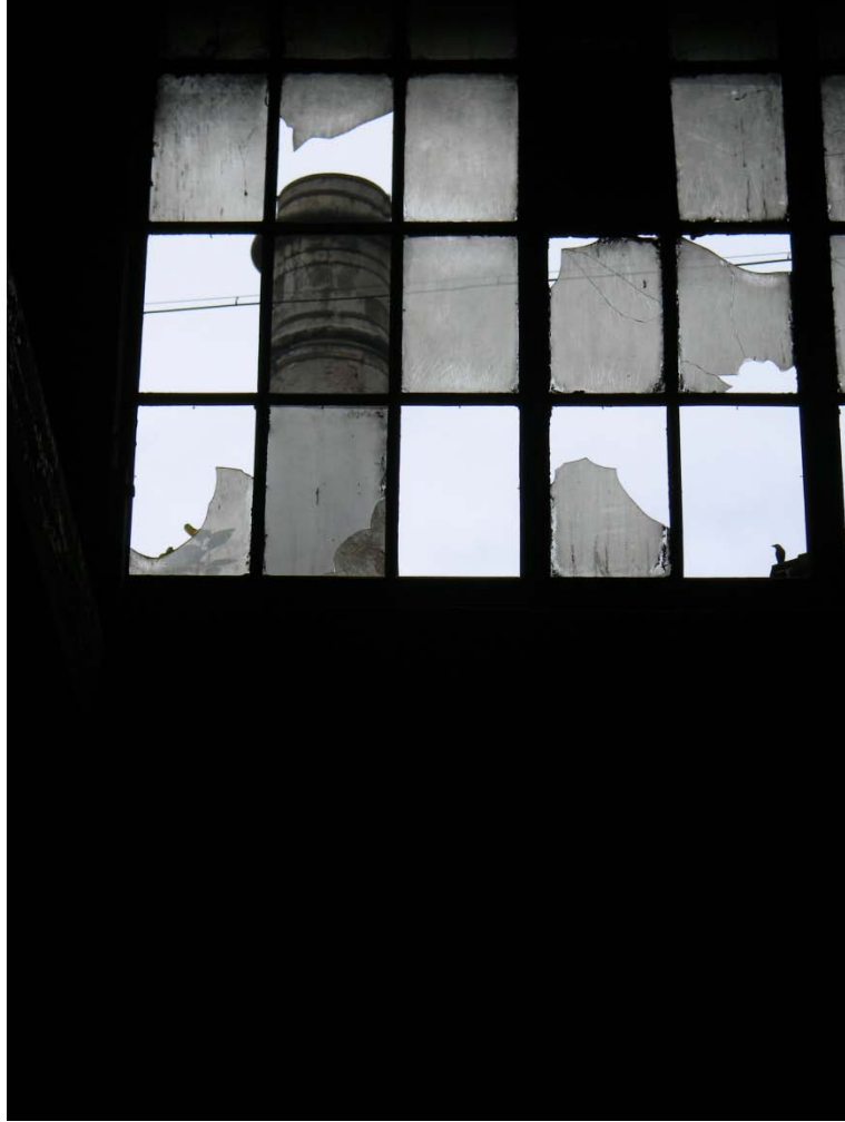
Figure 63: Mill Chimney (Author)
